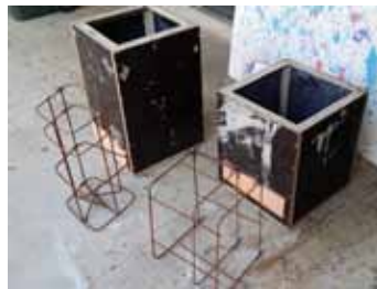
formwork for 2 sizes + reo cage.
